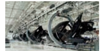
AFT electric monorail system
